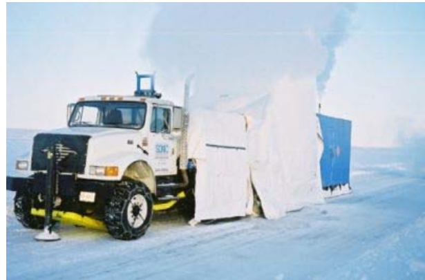
A sonic drill rig works around the clock on a frozen lake, drilling in the Canadian arctic to prove gas deposits.
