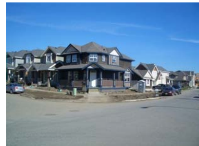
The small land footprint (above); the finished installation (below).
