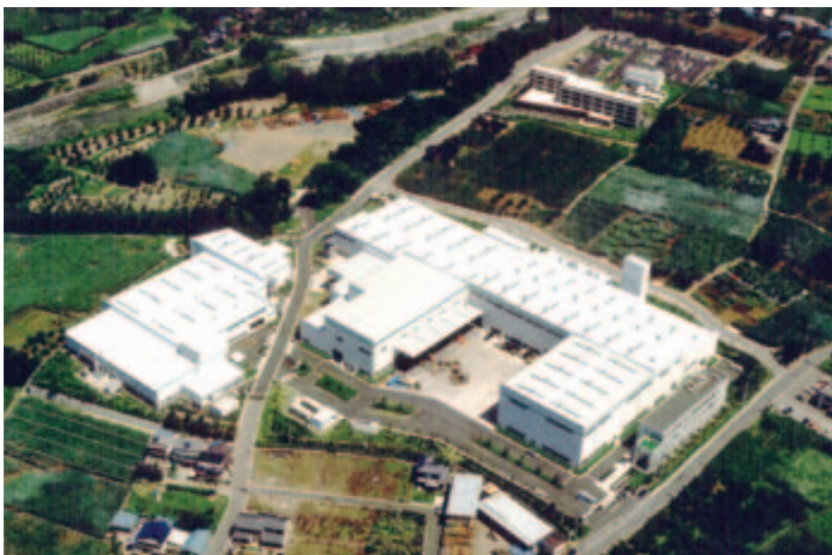
Aerial view of the Tone Boring building in Tokyo
