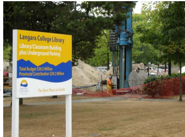
Speeding up the work at Langara, Vancouver.
